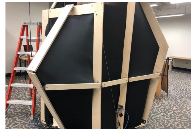
Figure 1: The outer shell of the pod made of plywood, metal, screws, bolts, nuts, peel and stick tiles and blackout fabric.
